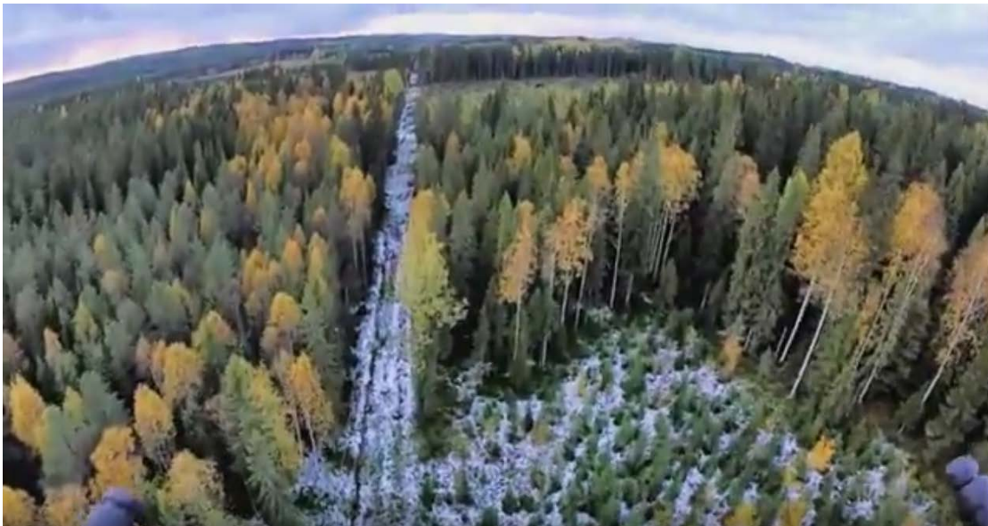
Power Line Corridor, UAV view
